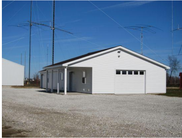
The K9CT Contest Station near Trivoli, Illinois (note two of the eleven towers visible on the left)
