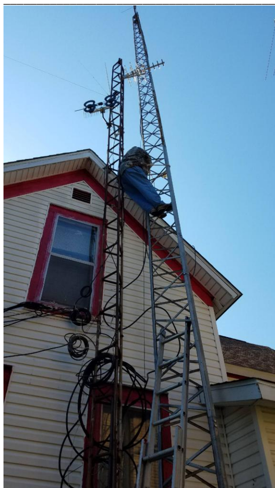
This is as high I will go up the tower. W3ML fixing his 160 meter dipole.
